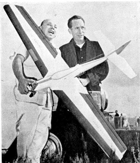
Dr. Ralph Brooke of Seattle and Orbit R/C proprietor Bob Dunham of Los Angeles with the former's World Championship winning R/C model at Genk, Belgium. Veco 45 R Engine, Orbit proportional controls, Glass Fibre fuselage.
